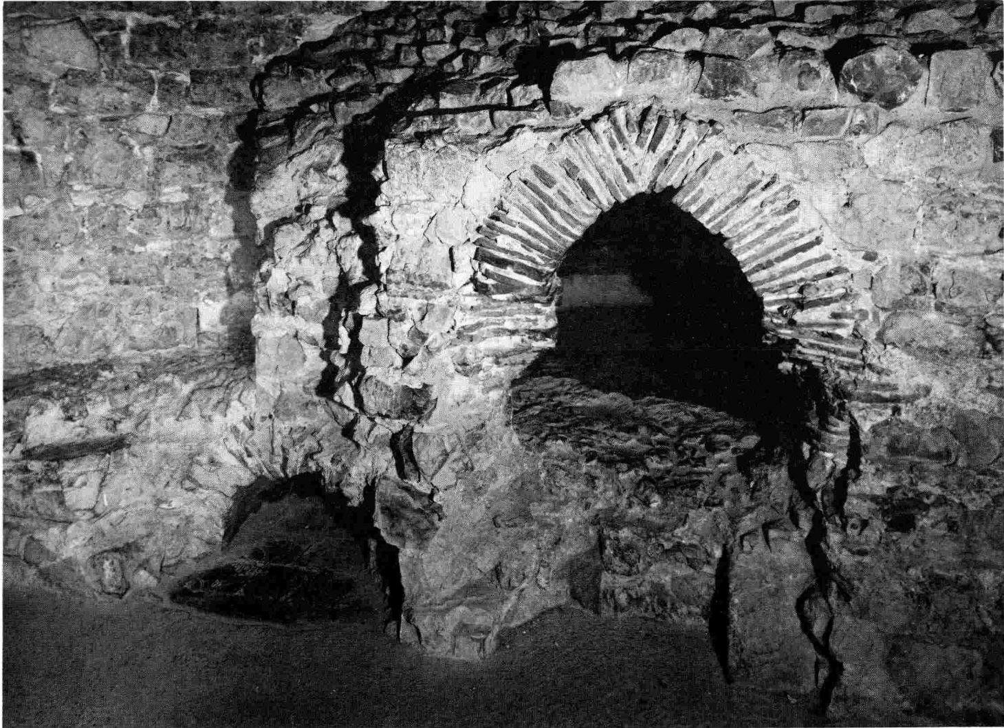
Orford Castle: the oven in the north turret, from the west, showing the decorated tile floor of the firing chamber (left) and the arch of roof tile sherds to the oven proper (right). P. Drury and E. Norton
